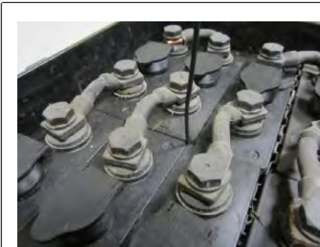
Set the temperature probe between the battery elements.
